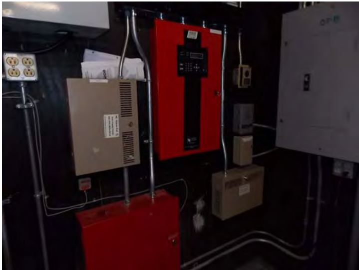
The central fire alarm control panel; it governs the common area detection and alarm devices.
