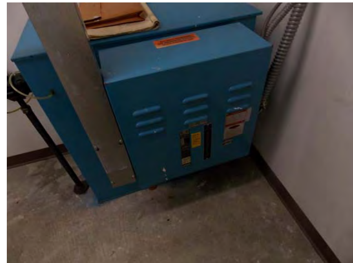
A view of the elevator hydraulic pump station.
