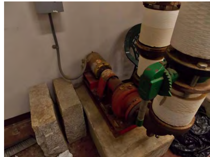
One of the hydronic circulating pumps.
