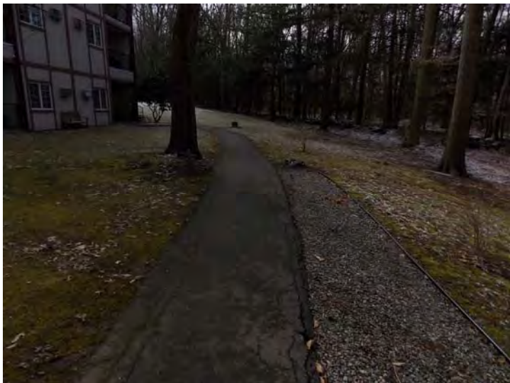
This is one of the asphalt-paved walkways; note the cracks along the right side.
