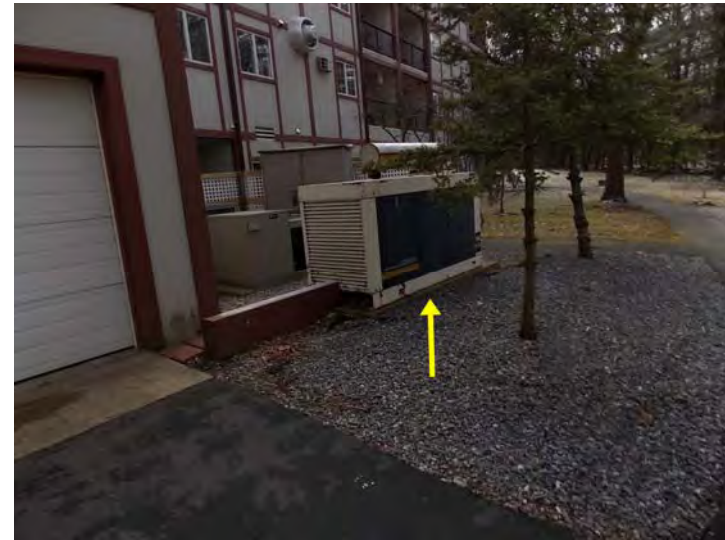
Emergency power is provided by this 100 kW generator.
