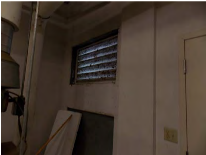
Fresh air for combustion in the boiler room is provided through this louvered opening.
