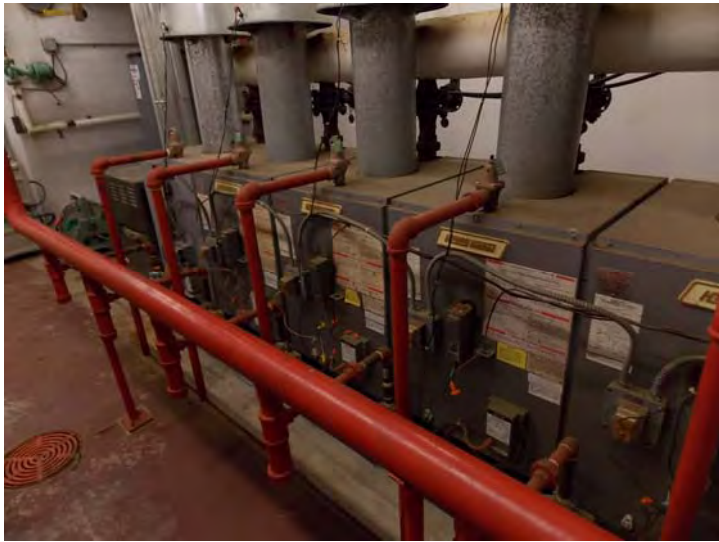
This is the boiler plant that produces the hydronic heat.
