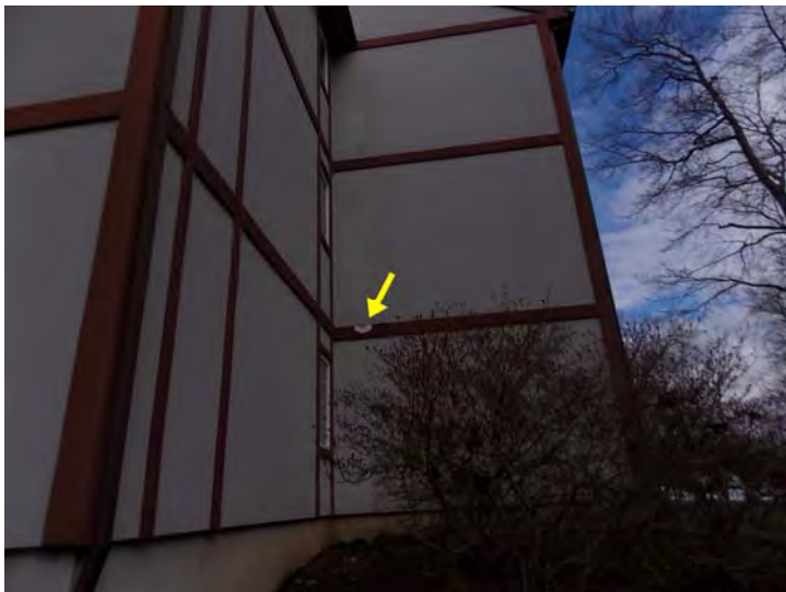
Most of the siding is synthetic stucco. The arrow is pointing to a damaged section.
