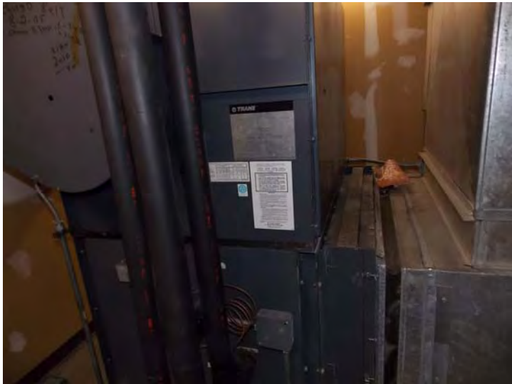
This is one of 2 air handlers, both which serve the common areas.
