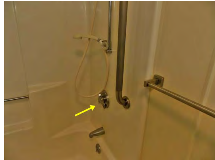
Bathtubs have an anti-scald mixing valve (arrow).
