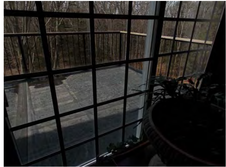
This roof deck is covered with a rubber membrane.
