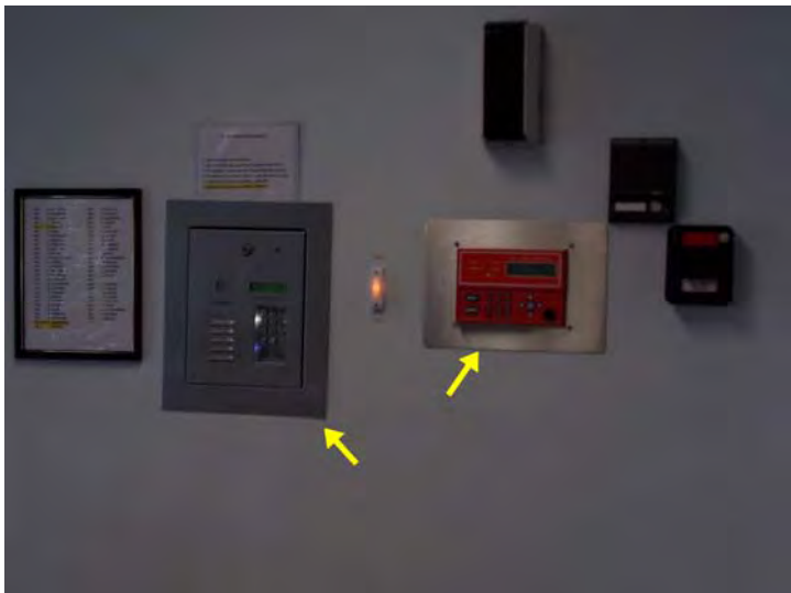
At the main entrance are the intercom panel (left) and the fire alarm annunciator panel (right).
