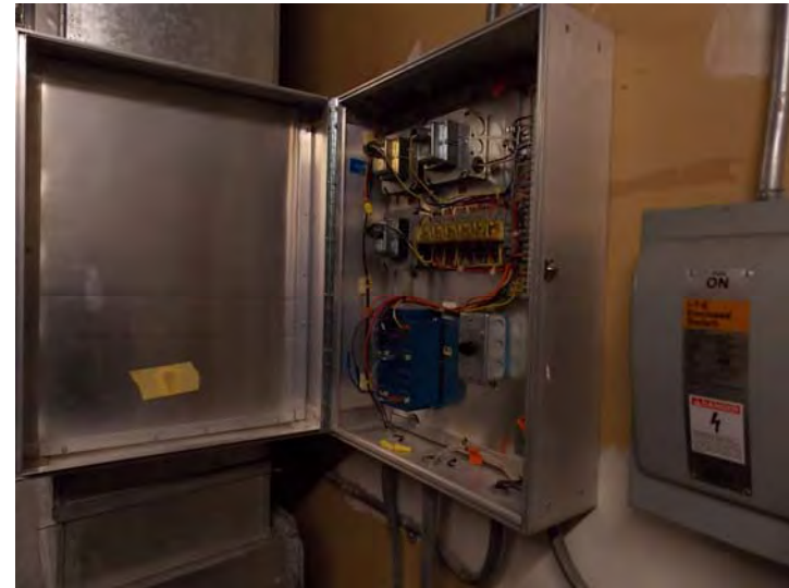
The controller for one of the air handlers.
