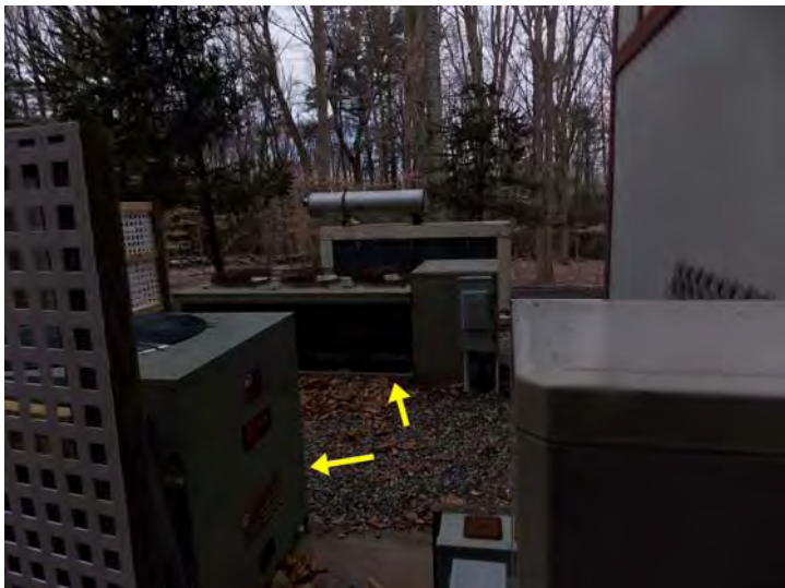
The air handlers have cooling coils from split DX air conditioning systems. The arrows point to the air-cooled condensers.
