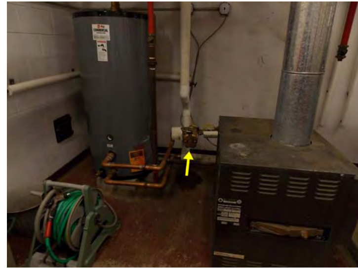
This dedicated DHW boiler (right) and storage tank (left) serve the common areas. The arrow is pointing to a DHW circulating pump.
