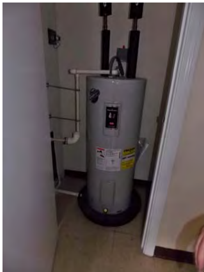
Each unit has an electric-heated DHW tank.
