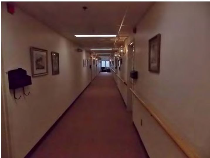
One of the common hallways, with T8 fluorescent lighting in ceiling, and LED wall sconces.
