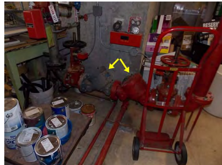
The fire sprinkler system has a backflow preventer, to keep stagnant sprinkler water from flowing back into the potable water.
