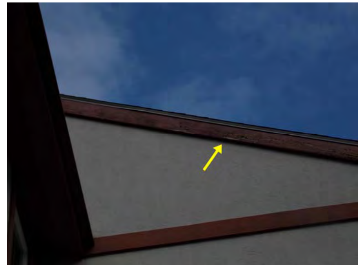
The wood trim along the roof line needs to be repainted.
