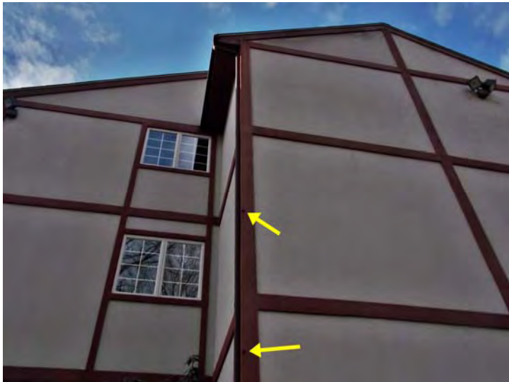
Isolated trim sections have been damaged by woodpeckers.
